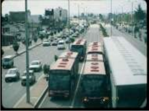
* Provision for Overtaking at BRT Station
